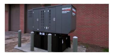
The NEC and NFPA compliant Generac diesel system has two outputs; one for life safety and the other for emergency power. The System features a sound attenuation package, keeping the noise produced by the generator down to a minimum. Since the American Red Cross is surrounded by residential homes, keeping noise to a minimum was an important feature.
